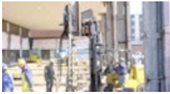
Auger Cast-In-Place Piles
